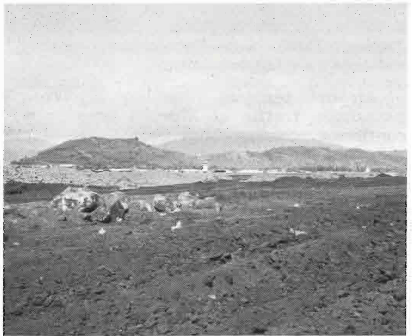
Construction underway on the north-south runway located at Lihue Airport.
