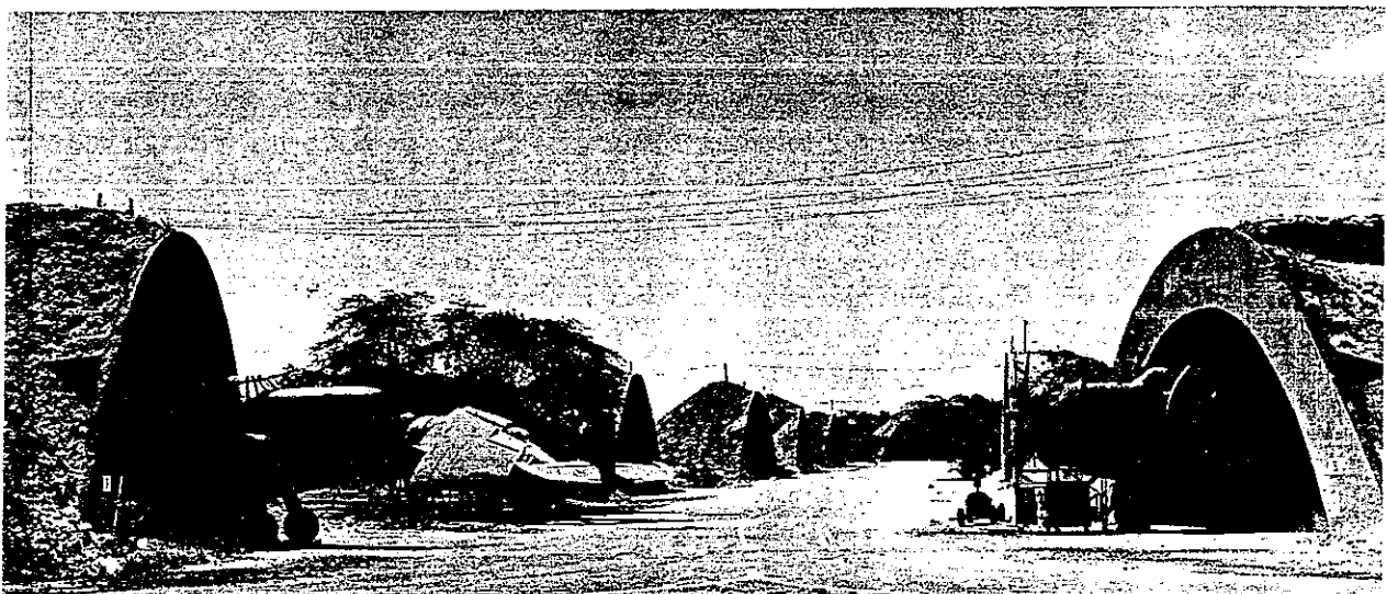
COVERED CONCRETE REVETMENTS, MARINE CORPS AIR STATION, EWA
