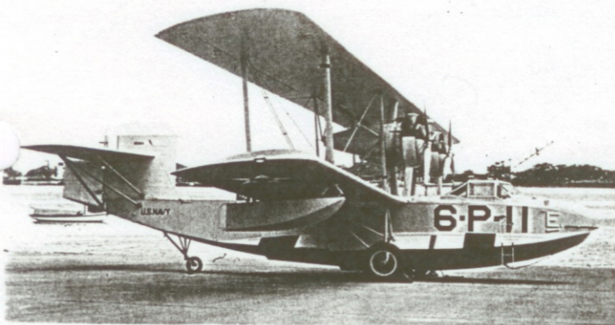
A PLANE OF SQUADRON VP-6F MODEL PM-1 BOAT TYPE SEAPLANE HAS GASOLINE CAPACITY FOR ABOUT ELEVEN HOURS DISTINGUISHING CHARACTERISTICS SINGLE VERTICAL RUDDER - COCKPIT GLASS ENCLOSED HULL PAINTED NAVY GREY ENAMEL TAIL SURFACES PAINTED BLUE
